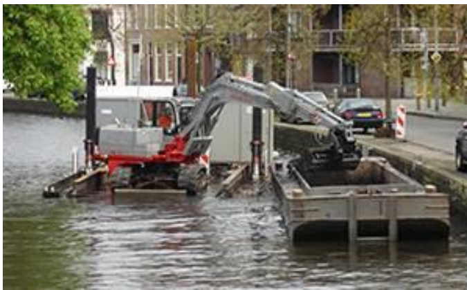
Photo: Excavator on a pontoon loading a barge
